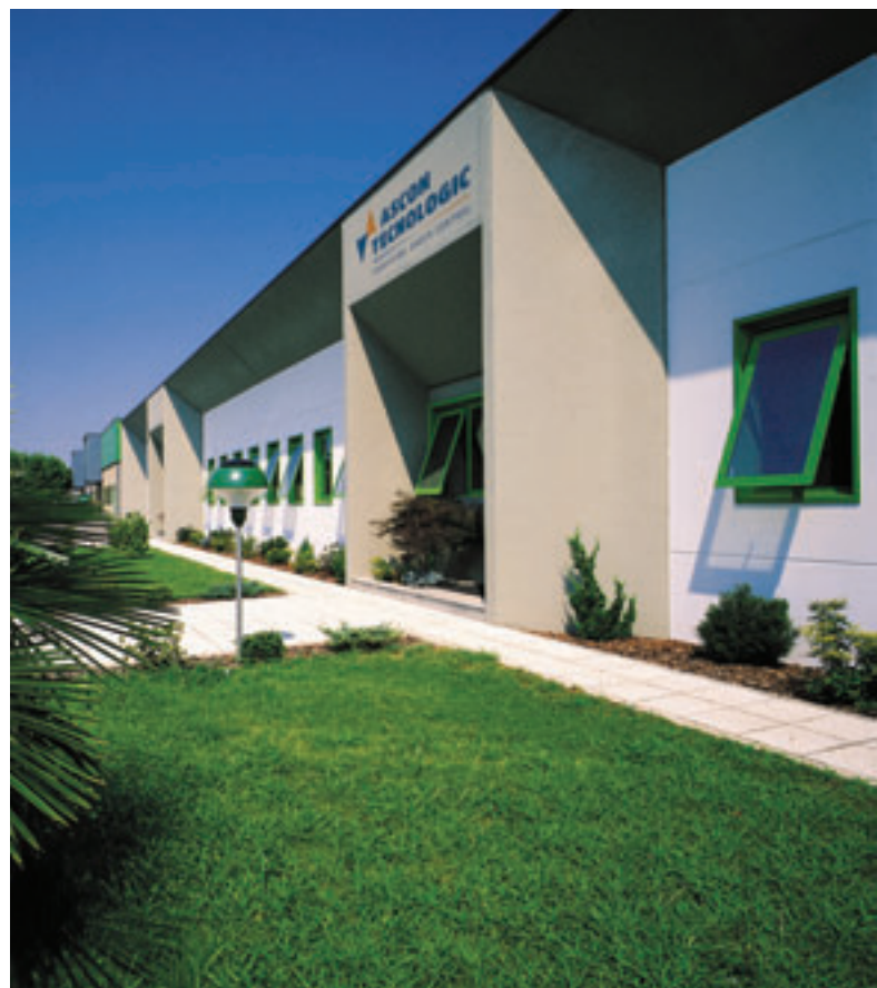
Headquarters, offices, R&D, Manufacturing unit, Vigevano (Italy).
