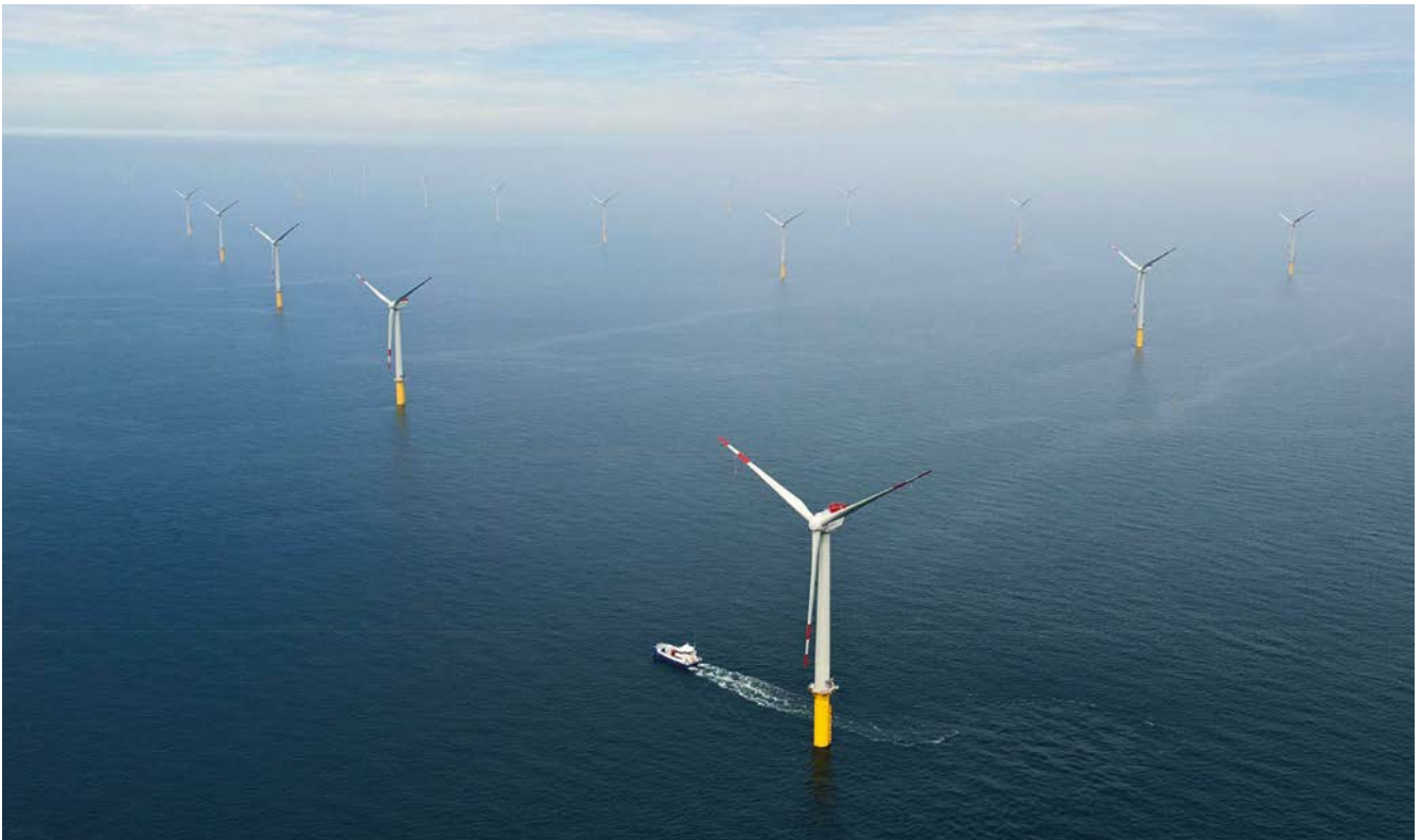
Borkum wind park project: 40 plants generate 750 gigawatts electricity annually on an area of 56 square kilometers. (Photo: Trianel GmbH/Jan Oelker)
